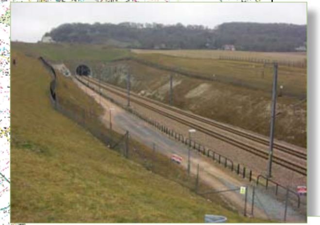
Photograph of HS1 tunnel entrance taken from a bridge across the Pilgrim Way in Kent.
