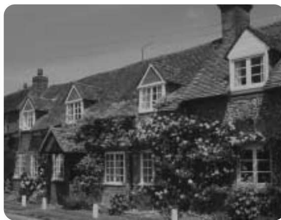
Brick and flint cottages at Turville (Z10)
